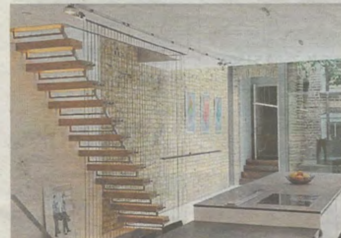
Unusual: LEDs are used to highlight the cantilevered oak staircase
